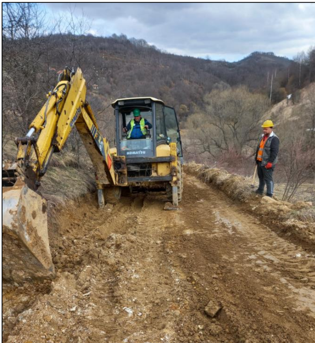
Figure 4. Access track construction at the southern end of Gradina.
