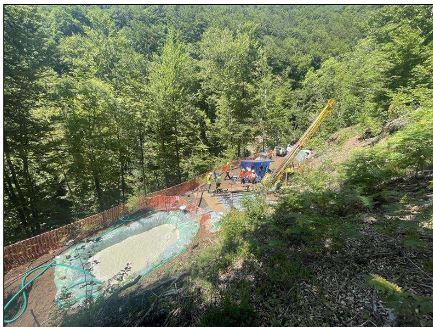
Figure 5. Diamond drilling rig 4
